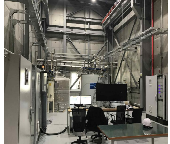
Linde L280 model : maximum condensing rate of 280 L/hour with total 8,000 L of LHe storage
